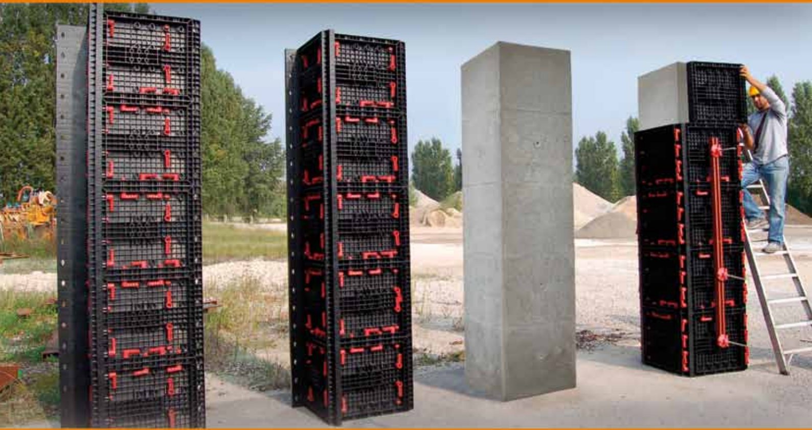
Reusable modular formwork for columns
